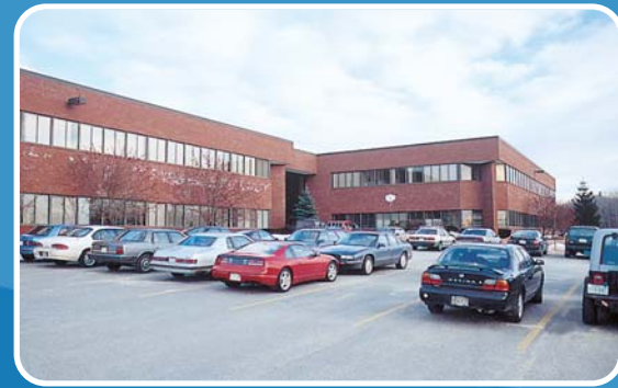
Transition Automation's state-of-the-art manufacturing facility in North Billerica, Massachusetts.
